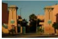
IMG21450 Entrance to parking area
