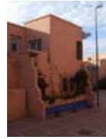
IMG21452 Façade of a two-family housing
